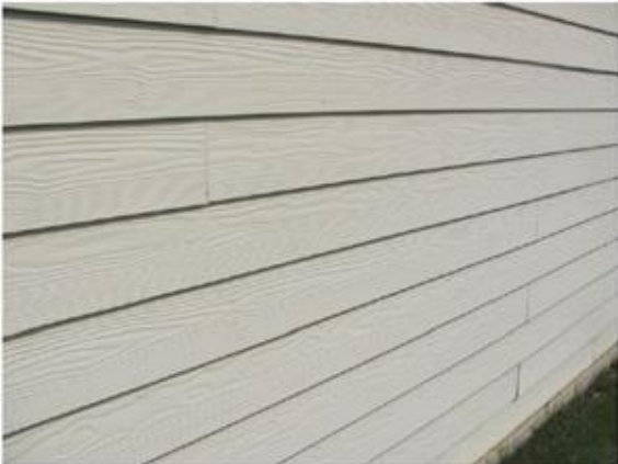
Fiber cement siding
