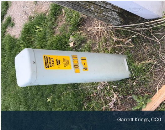
Pedestals / handholes
